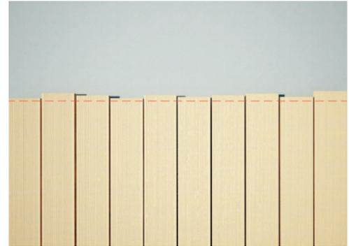
Prior to installation the deck boards, edge boards and edge skirts must be conditioned. Remove from their packaging and lay side by side 24hrs prior to fitting. Then trim to ensure they are all the same length.
