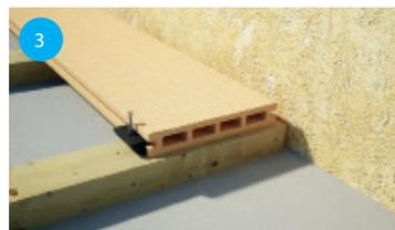
On every joist, position a hidden fixing clip into the groove of the first board and screw into position but do not tighten.
