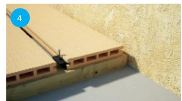
Slide the next deck board into position, locating the hidden fixing clip into its groove. This will set the gap between each deck board. Tighten the hidden fixing clip - but do not over tighten, use a low speed high torque setting on your electric screwdriver.
