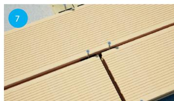
Where board ends meet allow an expansion gap (see expansion table) fit a second supporting noggins and fit a hidden fixing clip at the end of each board.
